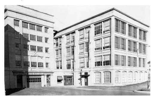
United Shoe Machinery designed the original buildings at Cummings Center with glass accounting for 75-90 percent of all wall space.
