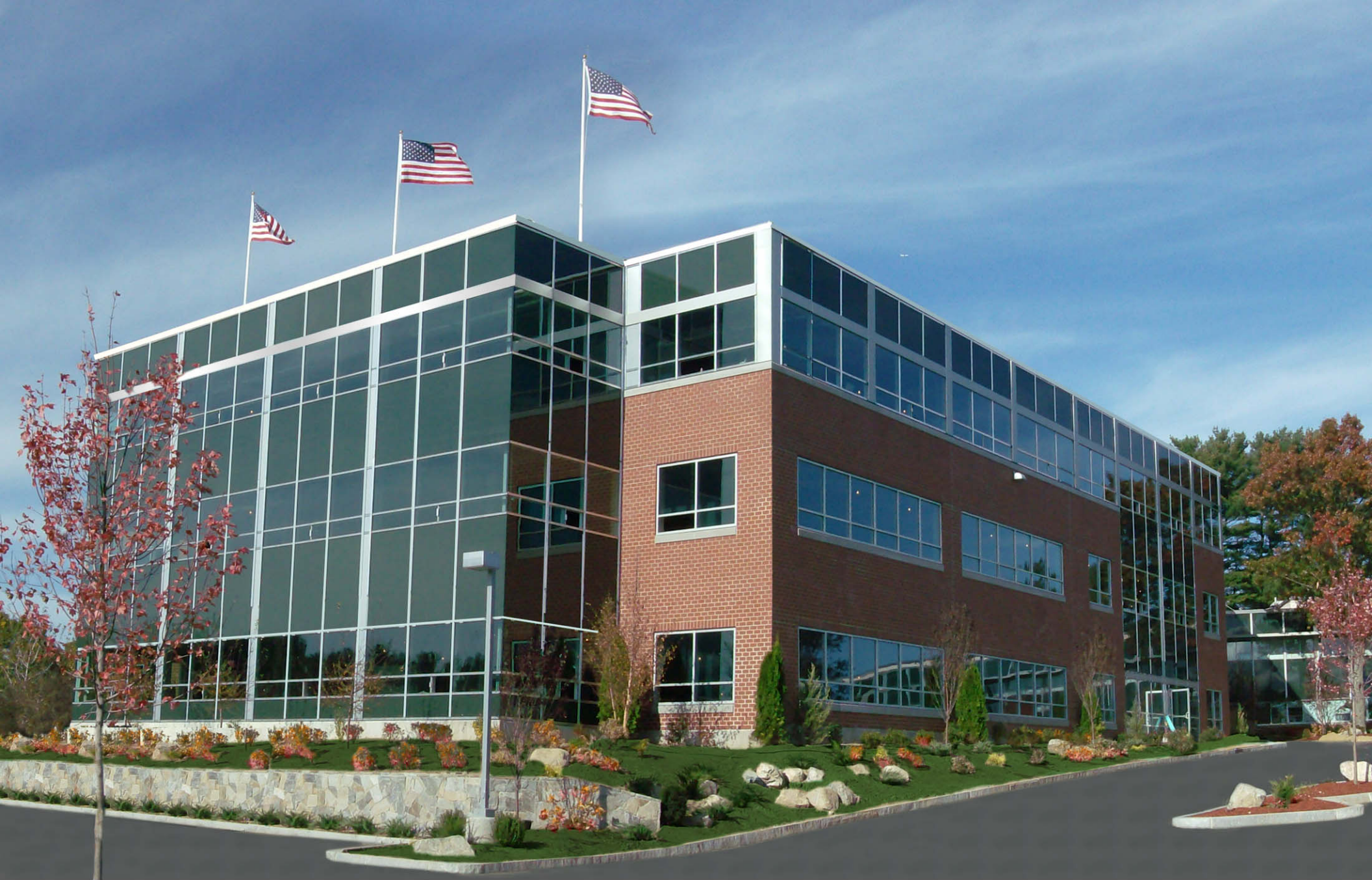
144 North Road, Sudbury
